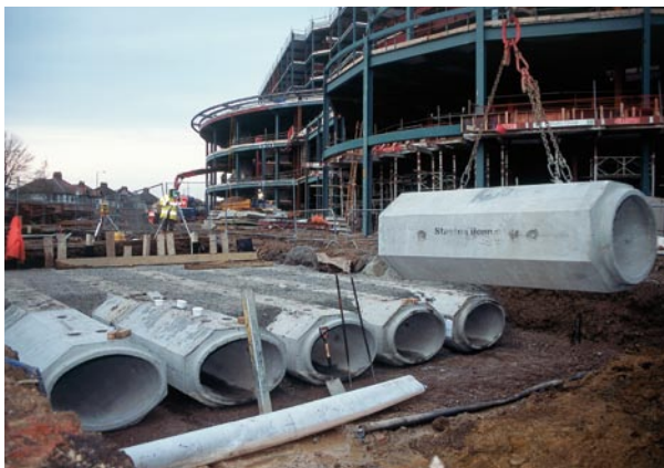
Elliptical tanks used for flood attenuation at Twickenham Rugby Stadium.
