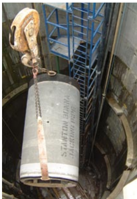
Pipe jacking is an excellent technology for reducing impact on the local environment as it leaves the ground undisturbed.
