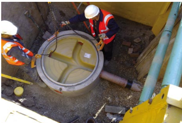
Precast manhole bases are watertight and save time on site.
